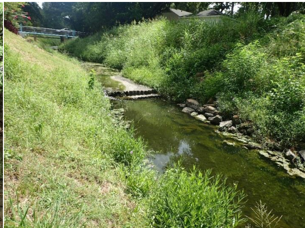
Figure 33. Concrete slab downstream of Rummel Creek Road
