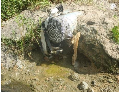
Figure 15. Outfall Tier II ID 035
