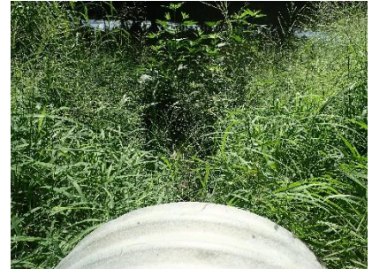
Figure 23. Outfall Tier No. 31
