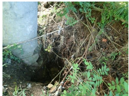
Figure 20. Outfall Tier II ID 052
