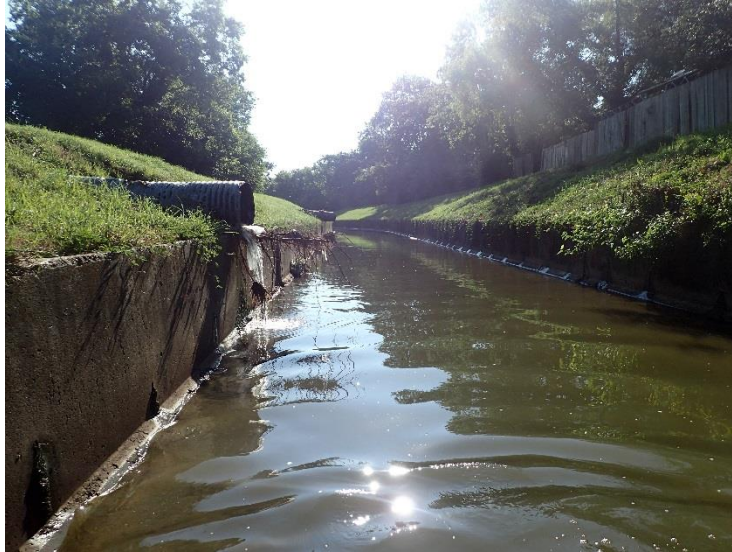
Figure 46. Outfall with dry weather discharge downstream of CRP monitoring station (sample 008)
