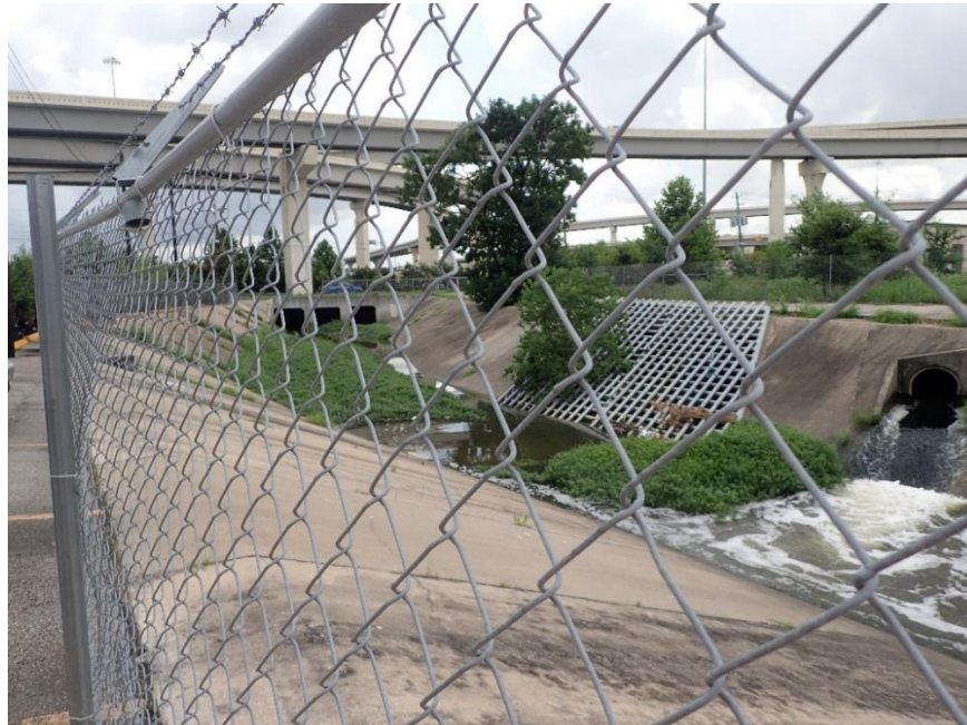
Figure 28. Stormwater detention outfall adjacent to plant nursery at southwest corner of I-10 and Beltway 8 intersection
