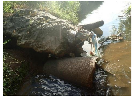
Figure 17. Outfall Tier II ID 040
