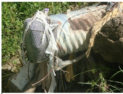
Figure 16. Outfall Tier II ID 035
