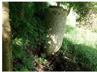
Figure 19. Outfall Tier II ID 052
