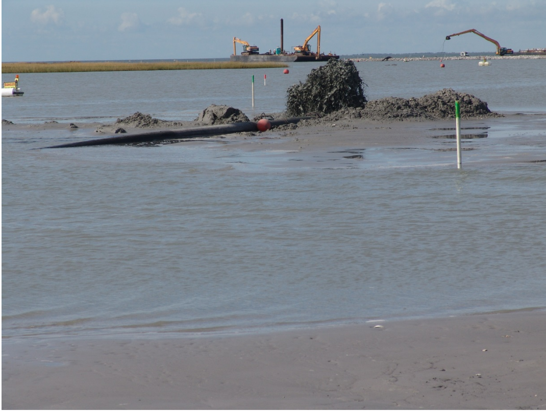
Figure 6. Hydraulic dredging of dredged material to construct marsh mound. Construction of rock breakwater in background.
