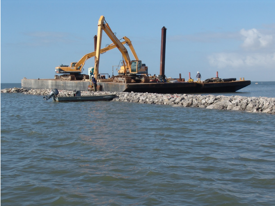
Figure 1. Construction of Breakwater. Excavators moving rock from barge to breakwater.
