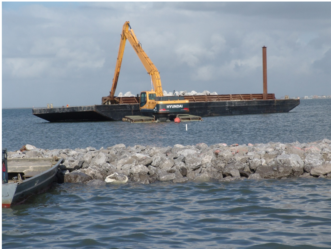
Figure 4. Smaller barge with shallower draft being brought to barge with excavator.
