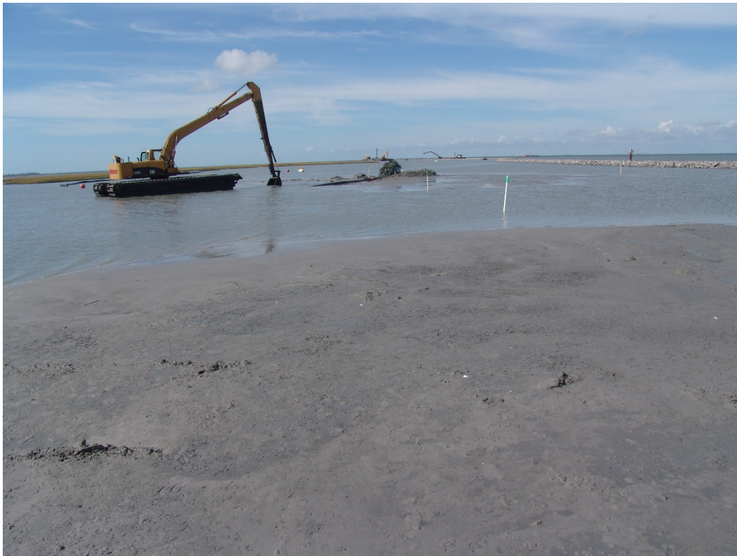
Figure 5. Hydraulic dredging of dredged material to construct marsh mound.
