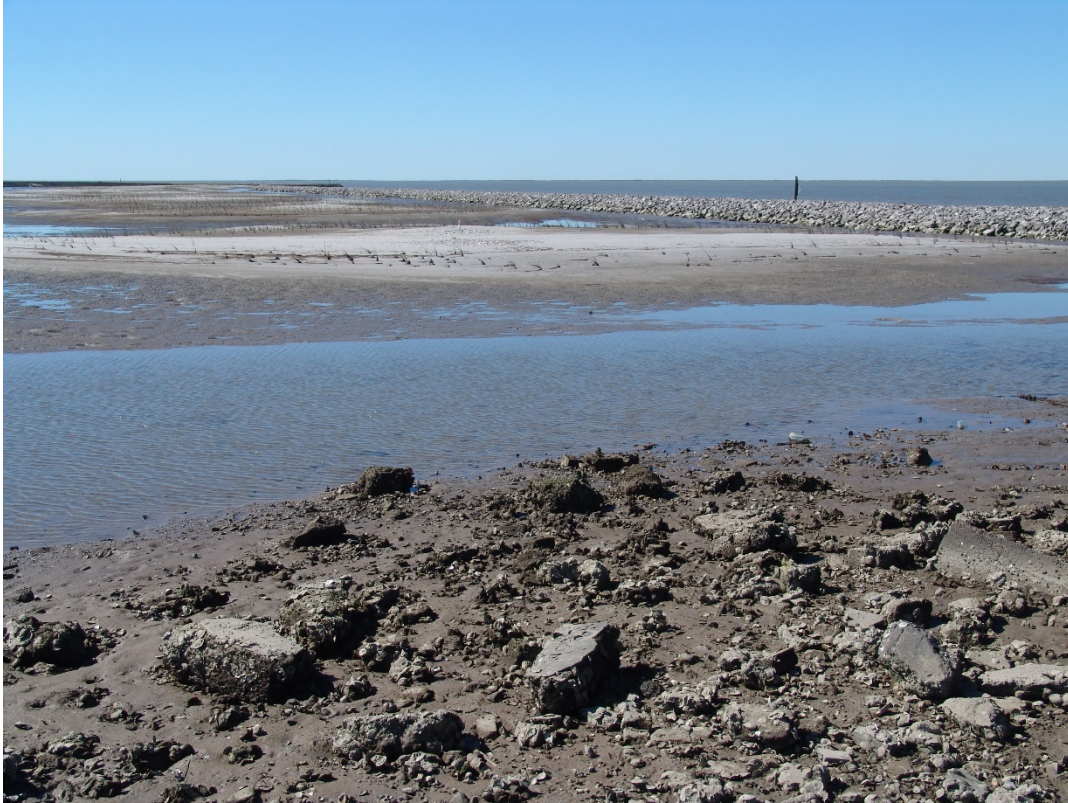
Figure 8. Completed marsh mounds. Rock breakwater in background.
