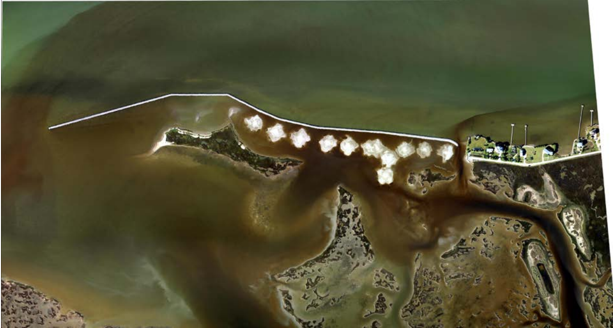
Figure 10. Aerial of completed project construction.
