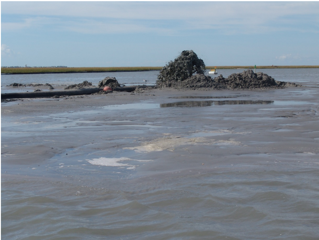
Figure 7. Hydraulic dredging of dredged material to construct marsh mound.
