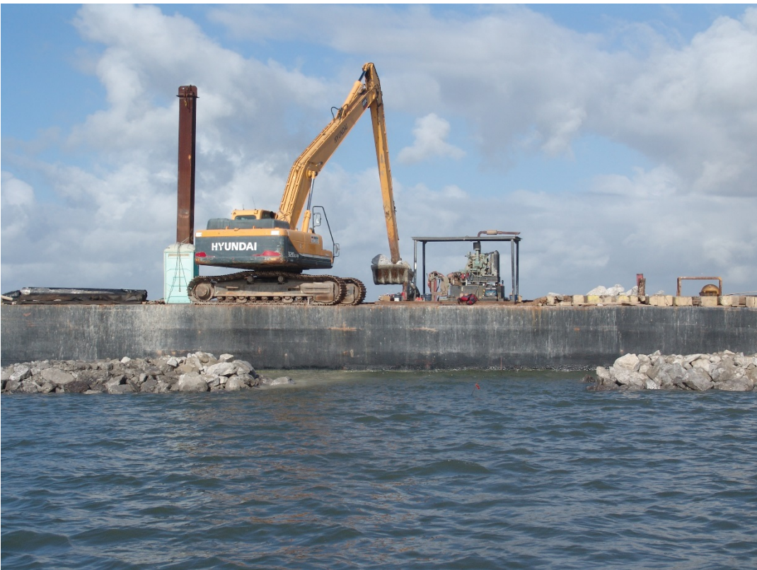
Figure 2. Construction of Breakwater. Excavator moving rock from barge to breakwater.
