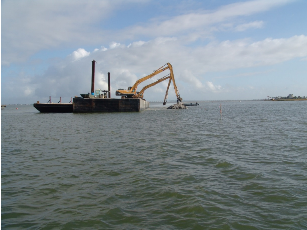
Figure 3. Construction of Breakwater. Excavators moving rock from barge to breakwater.
