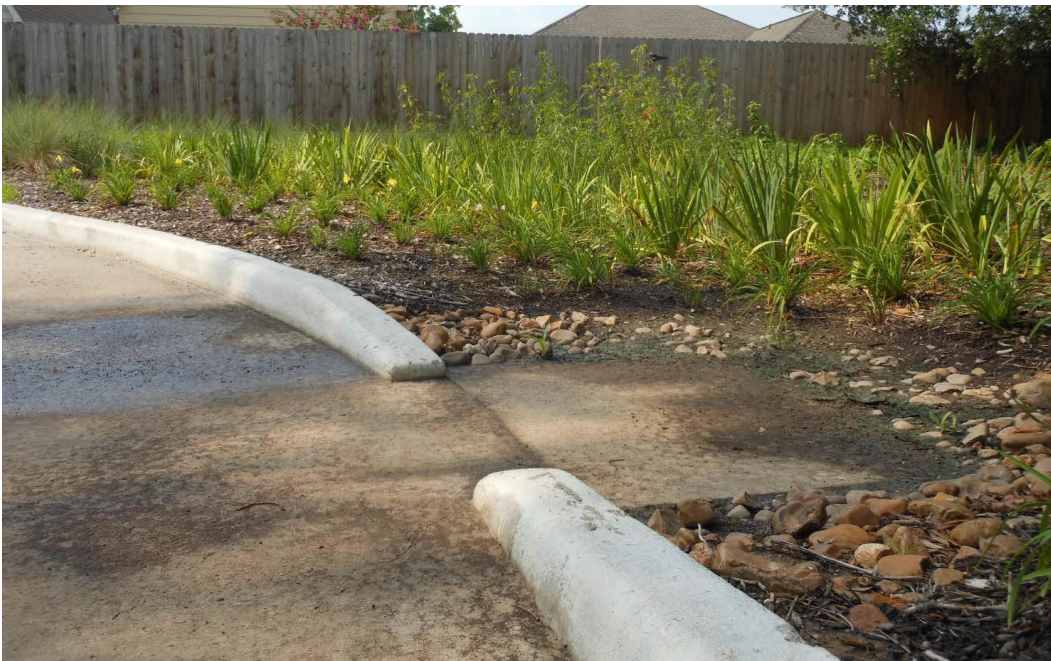
Figure 6: Curb cut that allows water from the parking area to flow into this rain garden for treatment
