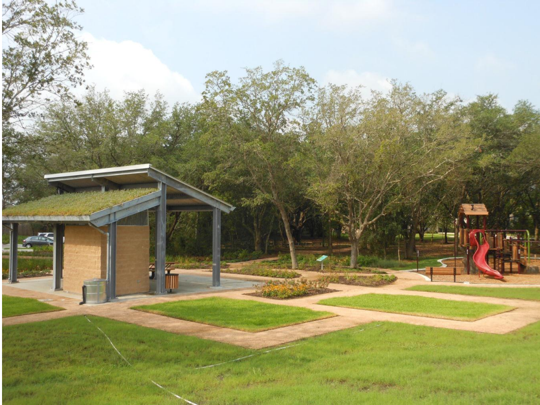
Figure 3: Green roof on the pavilion and WaterSmart Gardens
