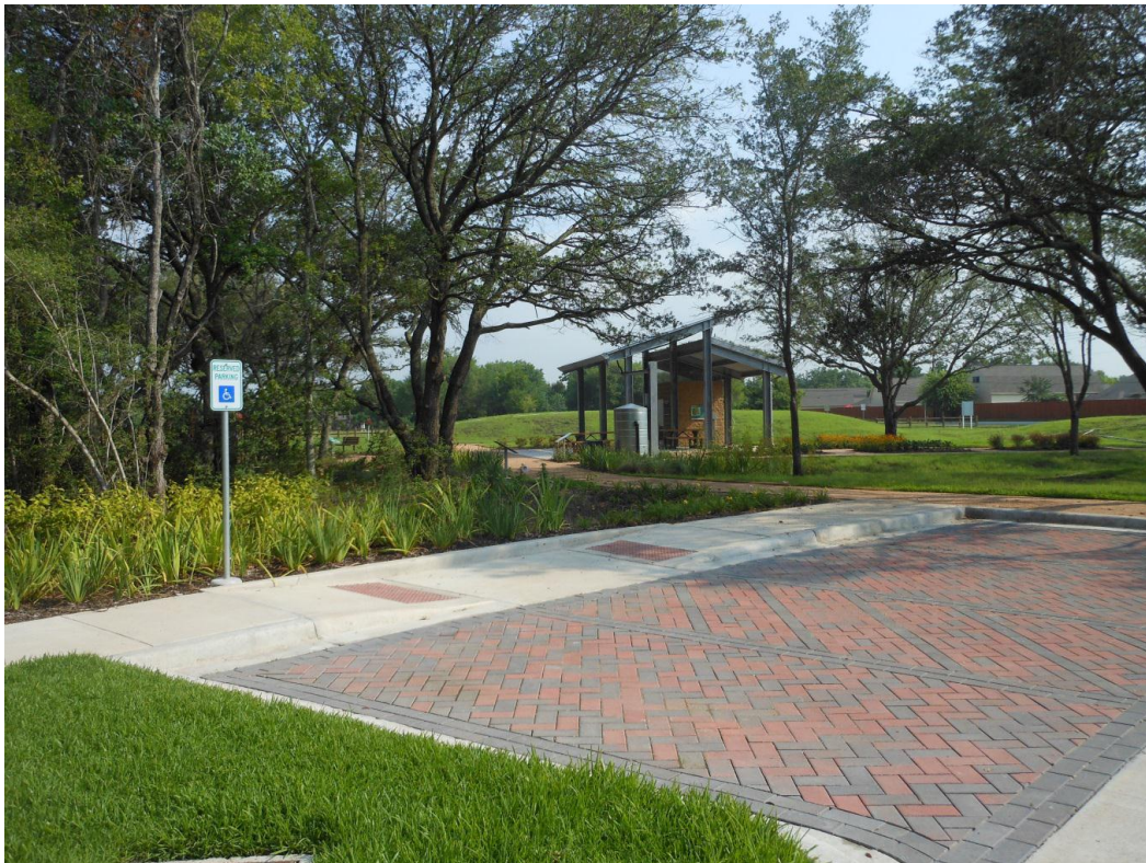
Figure 4: Pervious interlocking concrete pavers in the parking area
