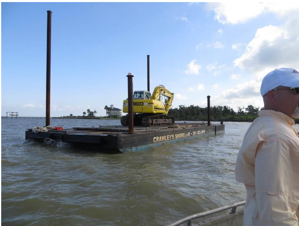
Trackhoe on barge used to deploy rip-rap
