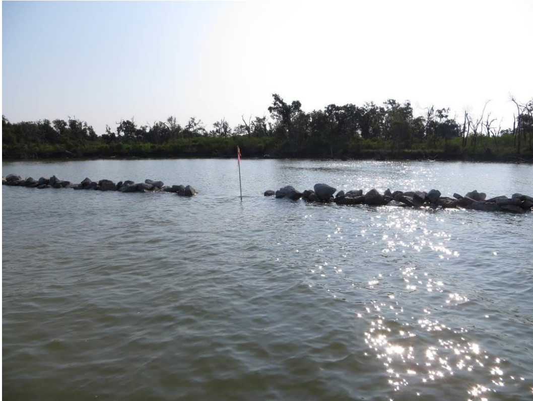
View of “low spot” in breakwater that allows ingress/egress of marine organisms
