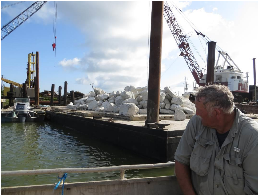
Rip-rap staged on barge and ready to transport to site
