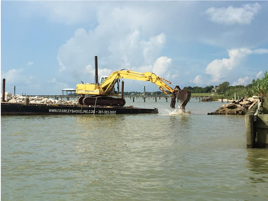
Figure 5. Start of construction of the southernmost section of rip-rap breakwater
