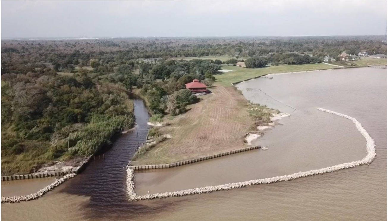
Figure 13. Aerial view of complete rip-rap breakwater and 300-foot oyster shell breakwater
