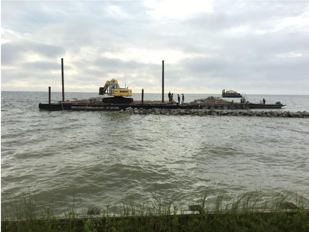
Figure 8. Ongoing construction of rip-rap breakwater
