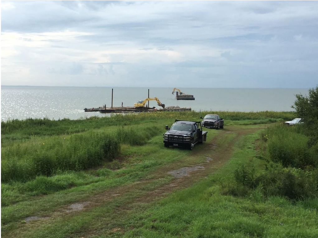
Figure 9. Ongoing construction of rip-rap breakwater
