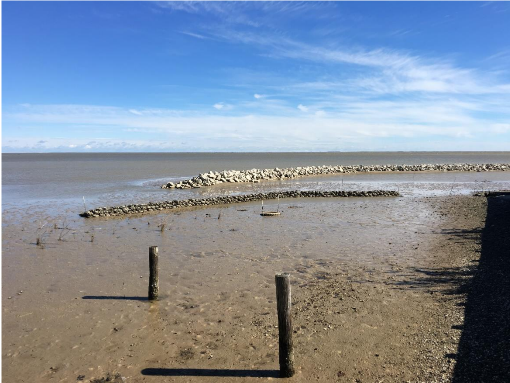
Figure 15. Oyster shell breakwater and rip-rap breakwater at low tide (December 2018)
