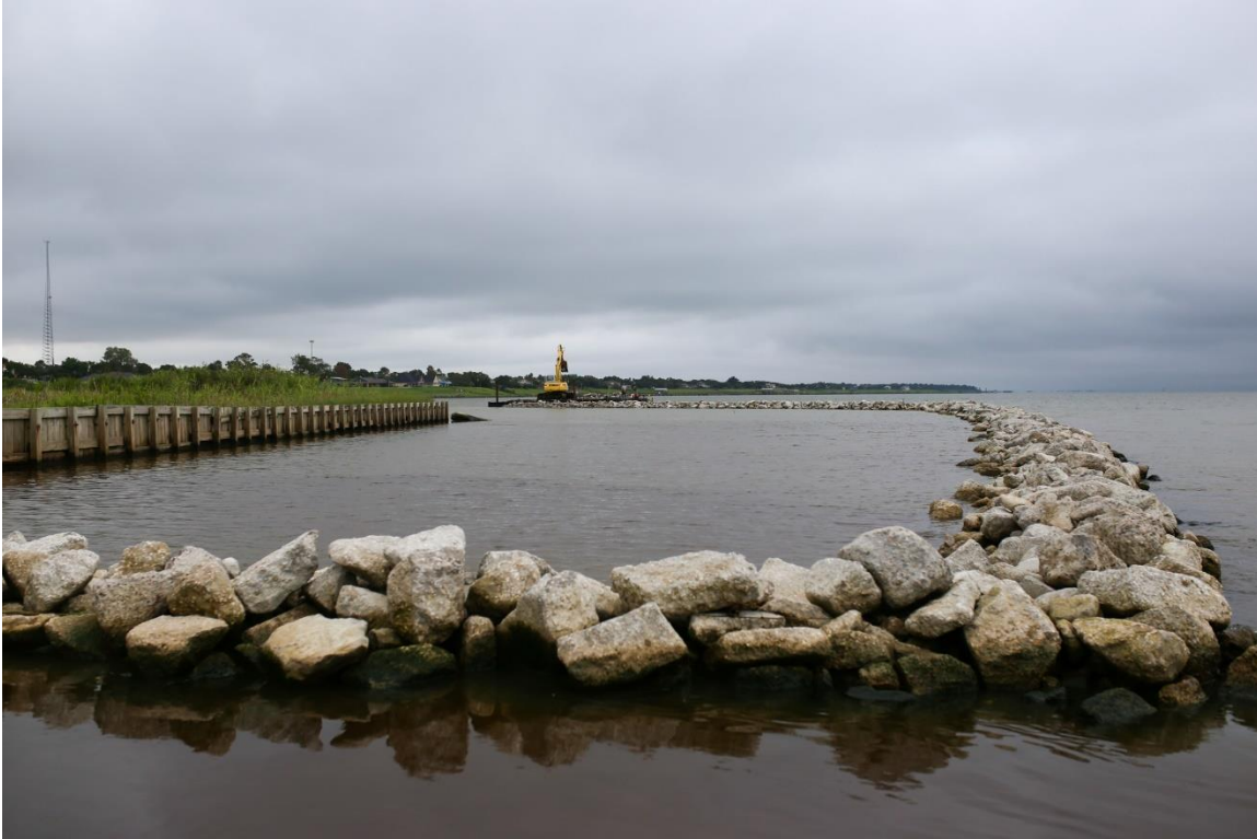
Figure 12. View of rip-rap breakwater looking north
