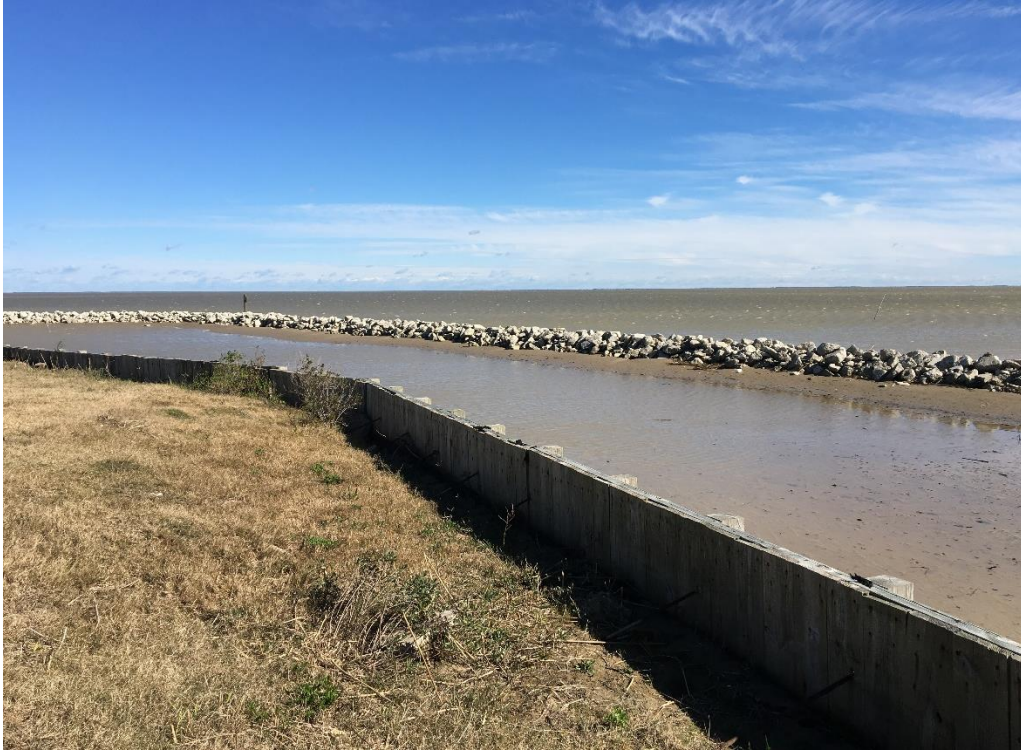
Figure 16. Rip-rap breakwater at low tide in December 2018, showing sediment accumulation directly behind the rocks
