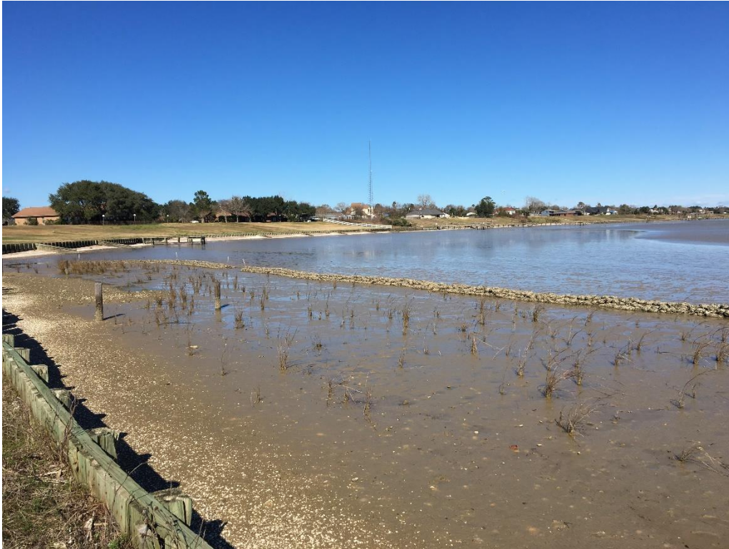
Figure 14. Oyster shell breakwater at low tide (December 2018)
