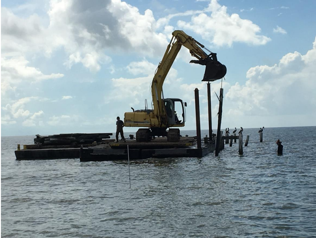
Figure 4. Removal of pier pilings/debris
