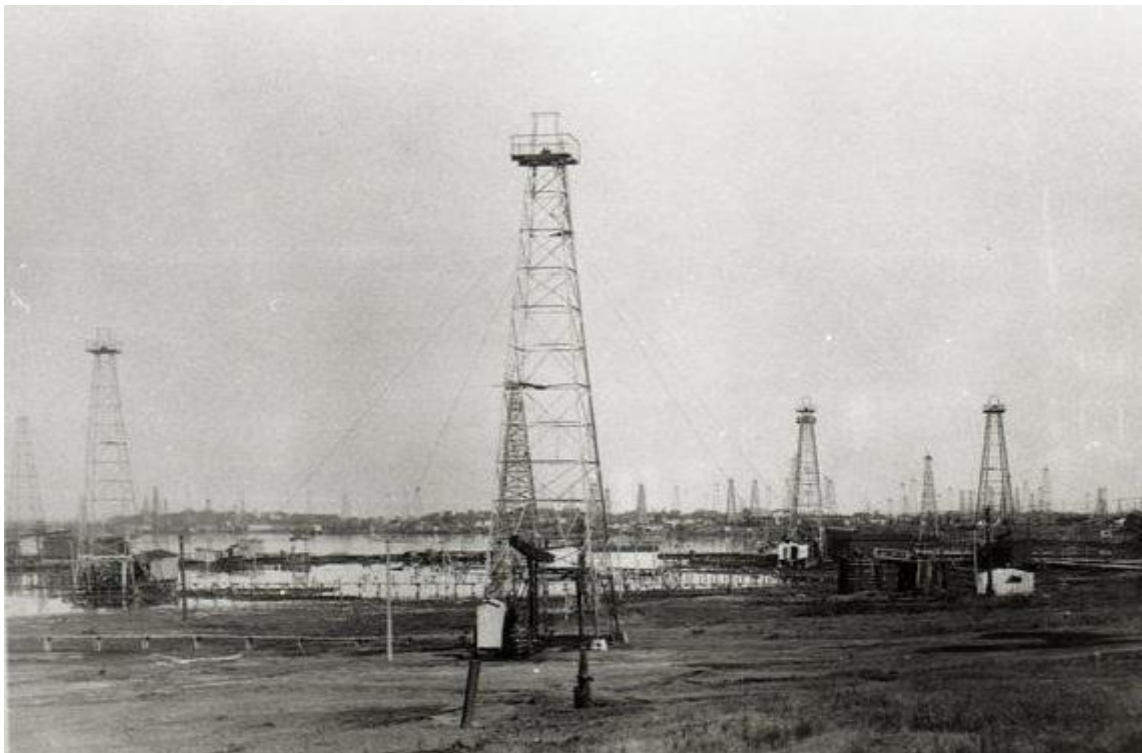
Figure 23 – Oil production in the Goose Creek oilfield (image courtesy of www.ourbaytown.com )
