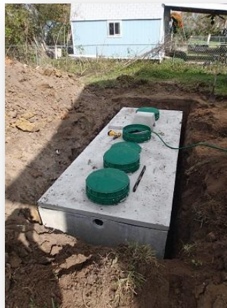
Figure 60 – OSSF being installed
