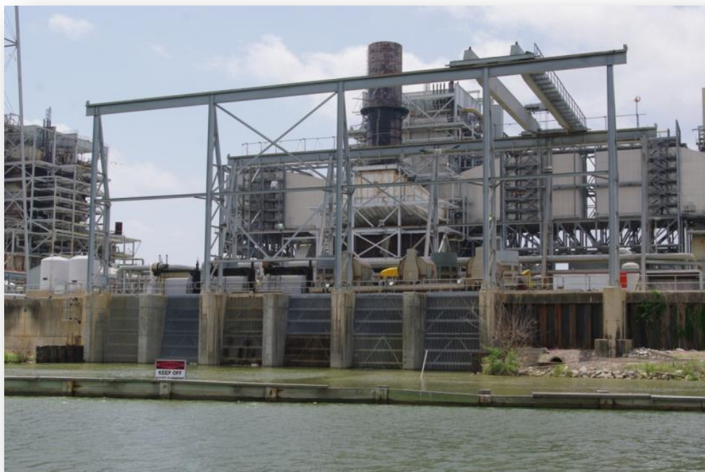
Figure 26 – Water intake at NRG Cedar Bayou Generating Station
