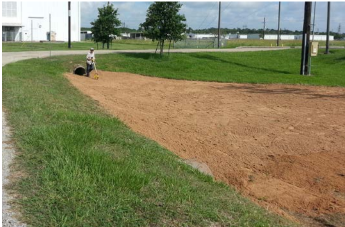
Preparation of the basin prior to planting.
