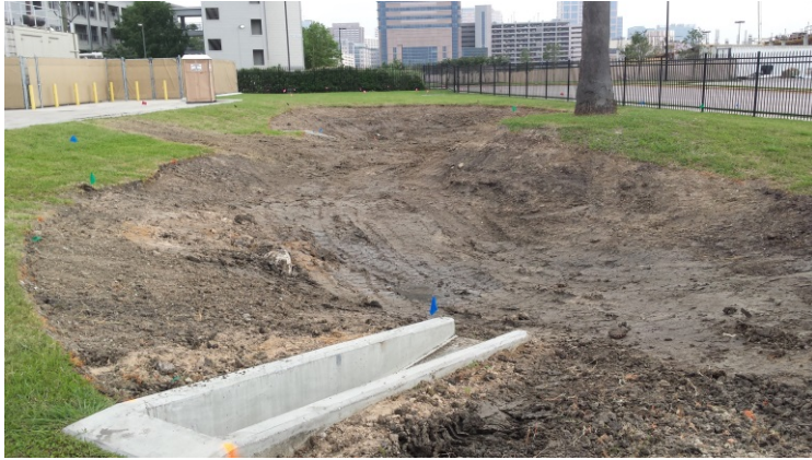
Completed fine grading of the MSF site.
