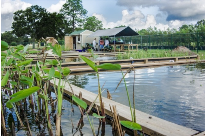
Ponds in the Exploration Green stormwater wetland nursery are shallow on-grade tanks formed by a lumber frame supporting a pond liner.
