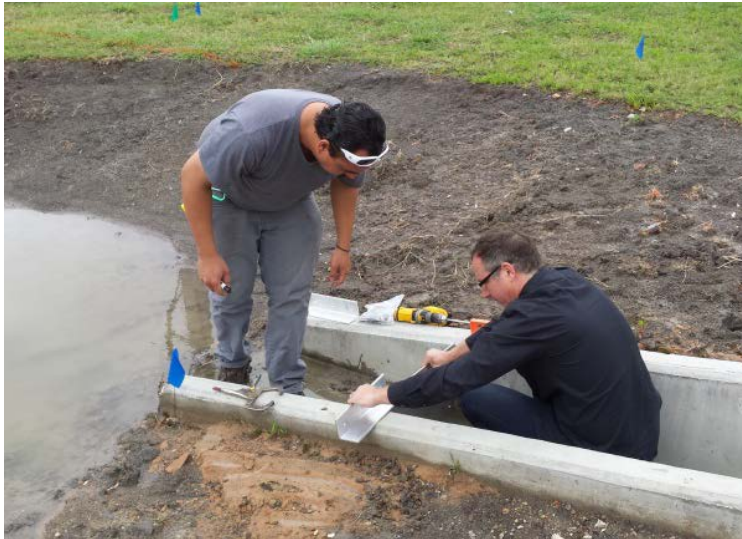
Weir installation at the MSF site.
