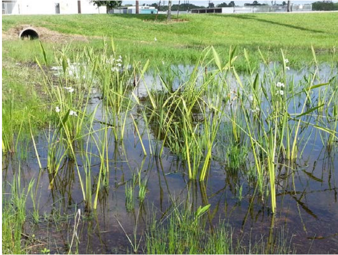
The wetlands, planted with species collected from ditches on the JSC campus, show signs of establishment one month after planting.
