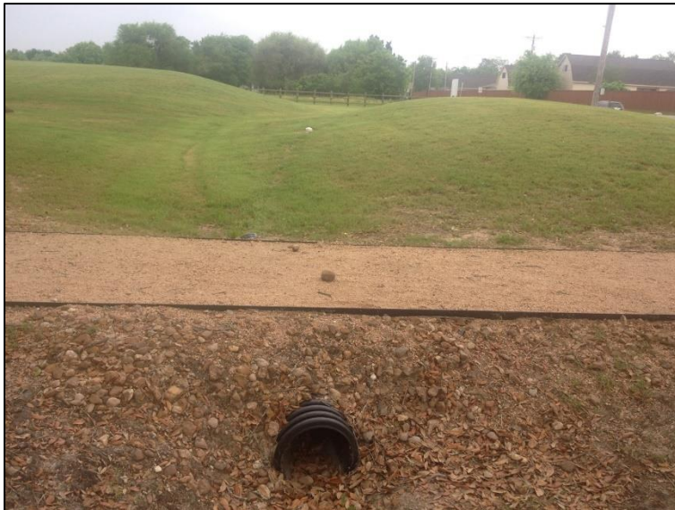
Figure 3. Bioswale vegetated with turf grass. Sampling point for this BMP is the pipe pictured.
