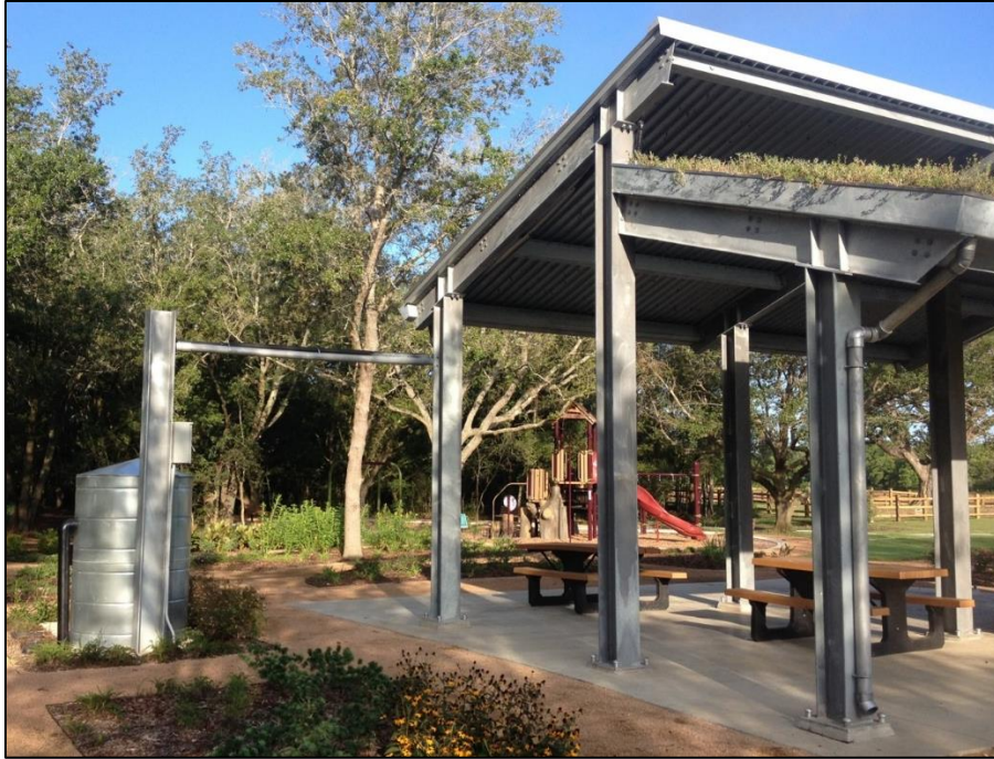
Figure 4. Pavilion at GFWP, the roof is split into two sections, allowing for both a green roof and rainwater harvesting practices on the same structure.
