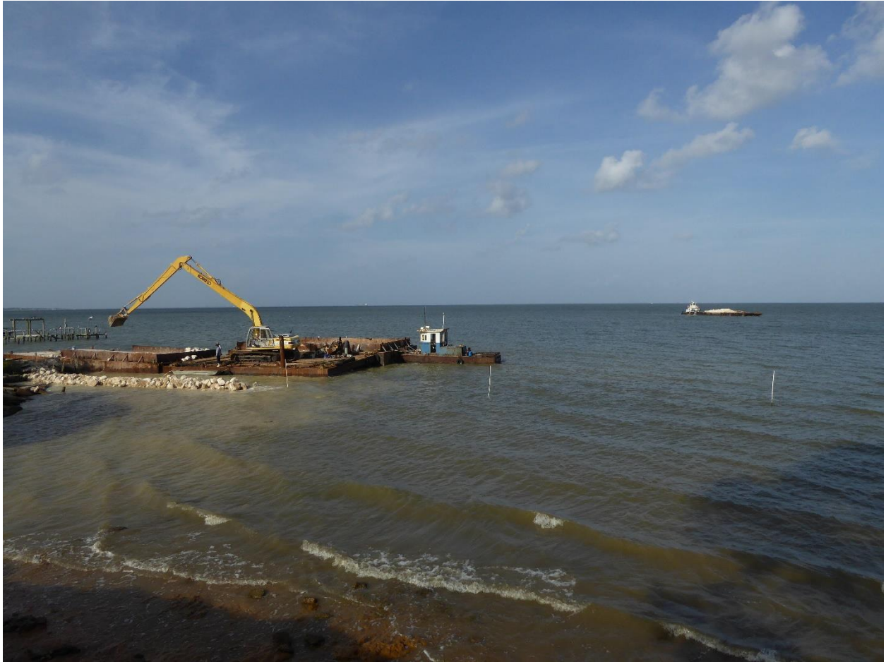
Figure 6: Construction along northern property line. Background: Barge bringing additional rip-rap
