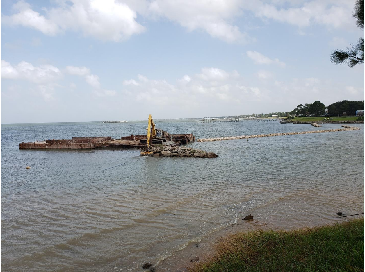
Figure 9: Removal of large concrete debris pile
