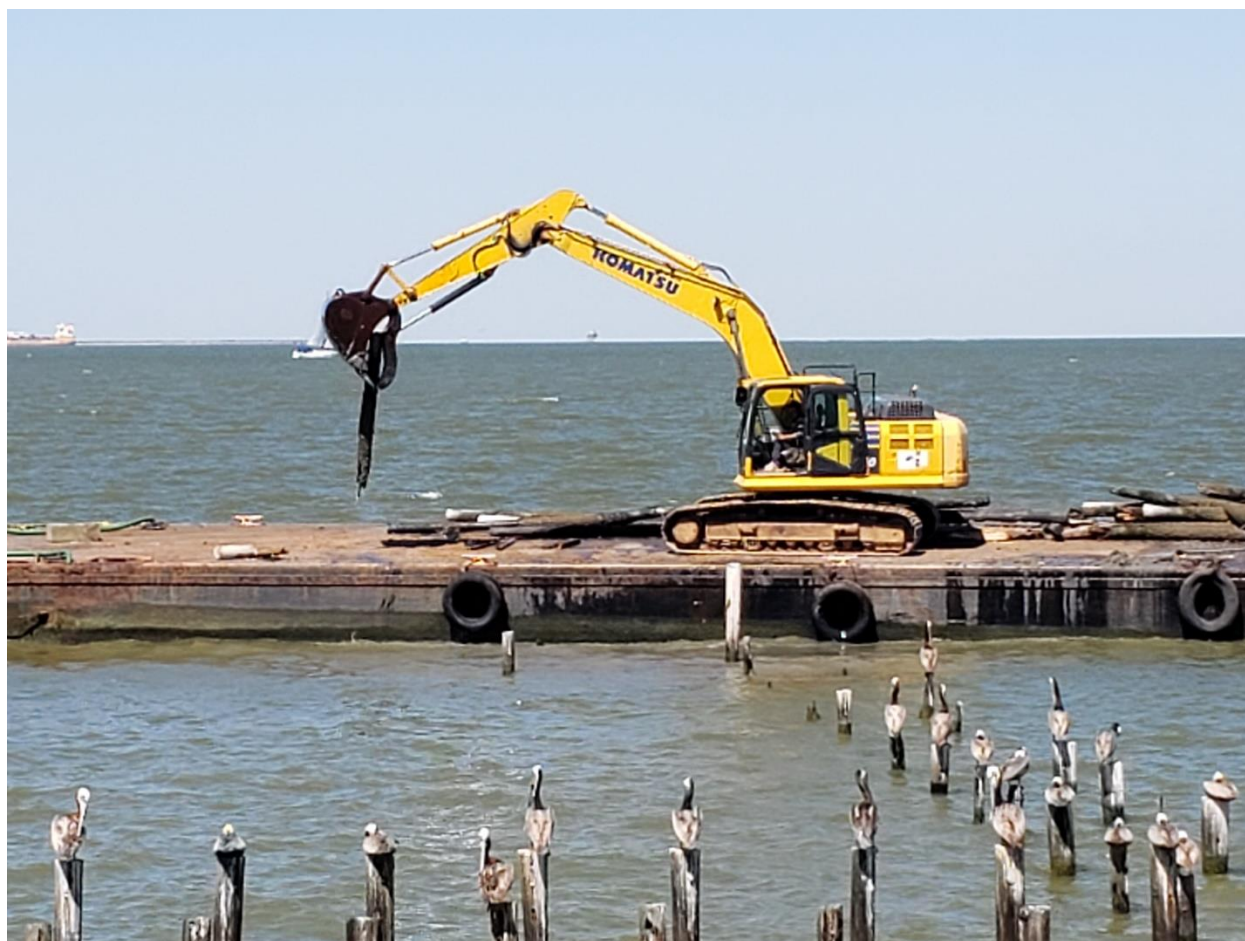
Figure 2: Derelict piling removal in process
