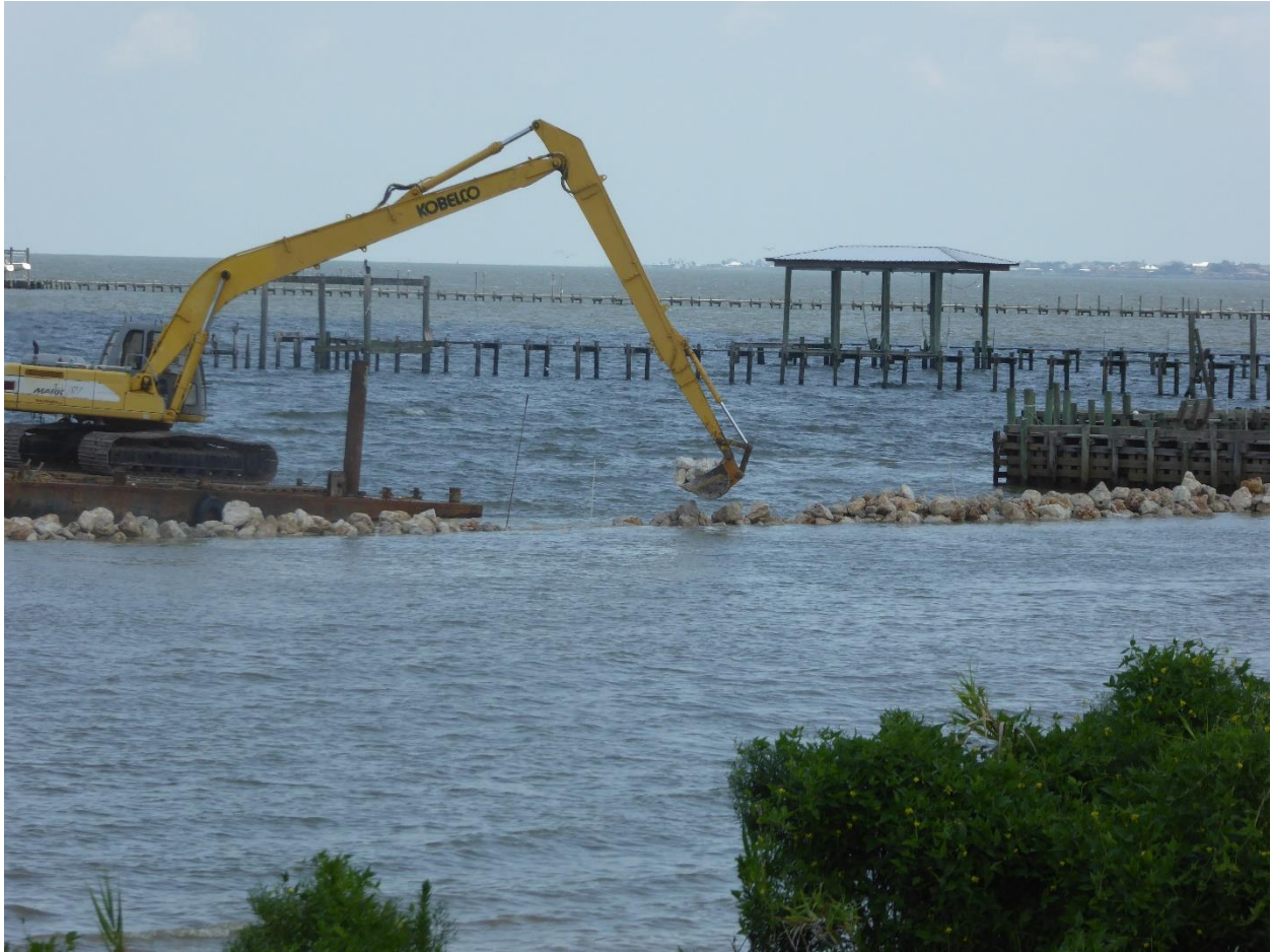
Figure 4: Day 1 of breakwater construction
