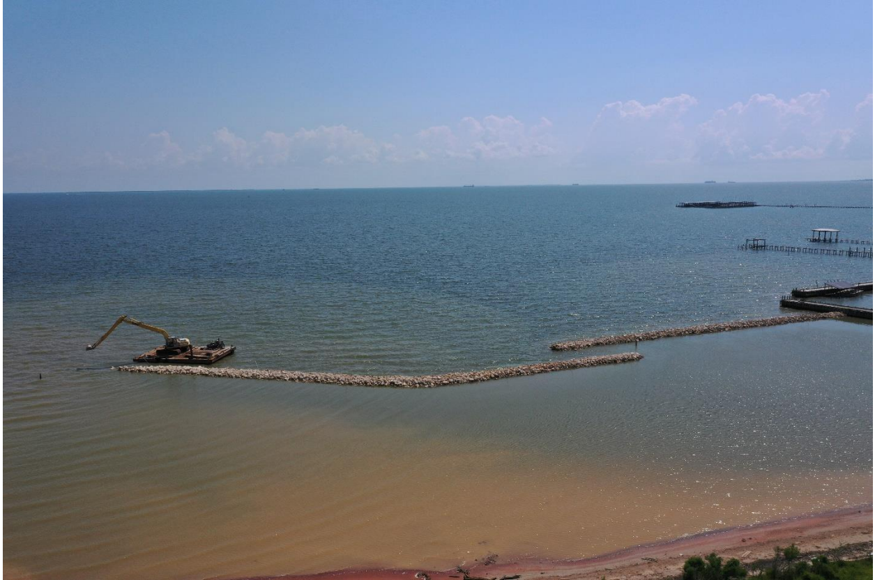
Figure 5: Breakwater at approximately 50% completion
