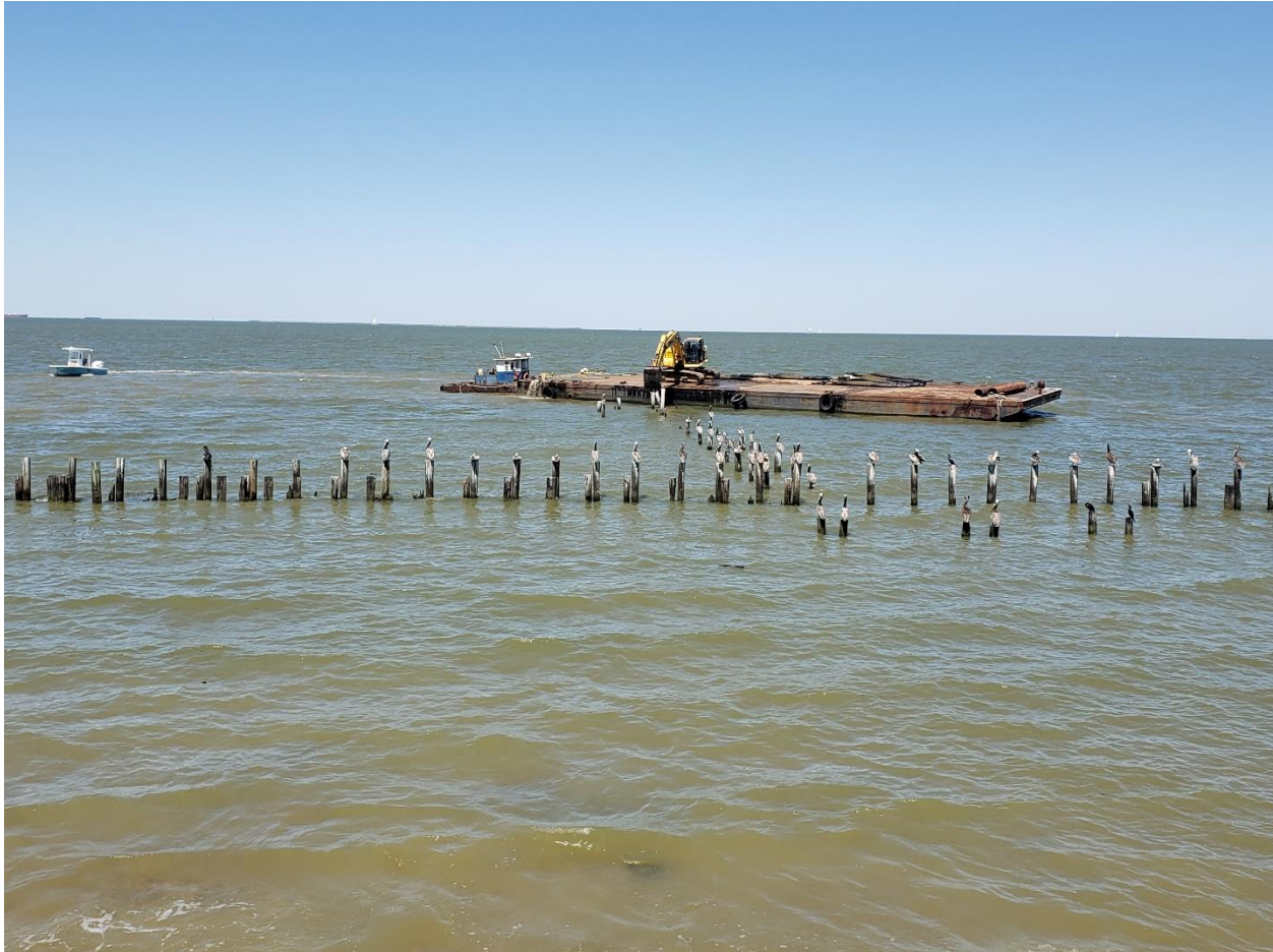
Figure 1: Equipment mobilizes onsite to remove derelict pier and bulkhead pilings and debris
