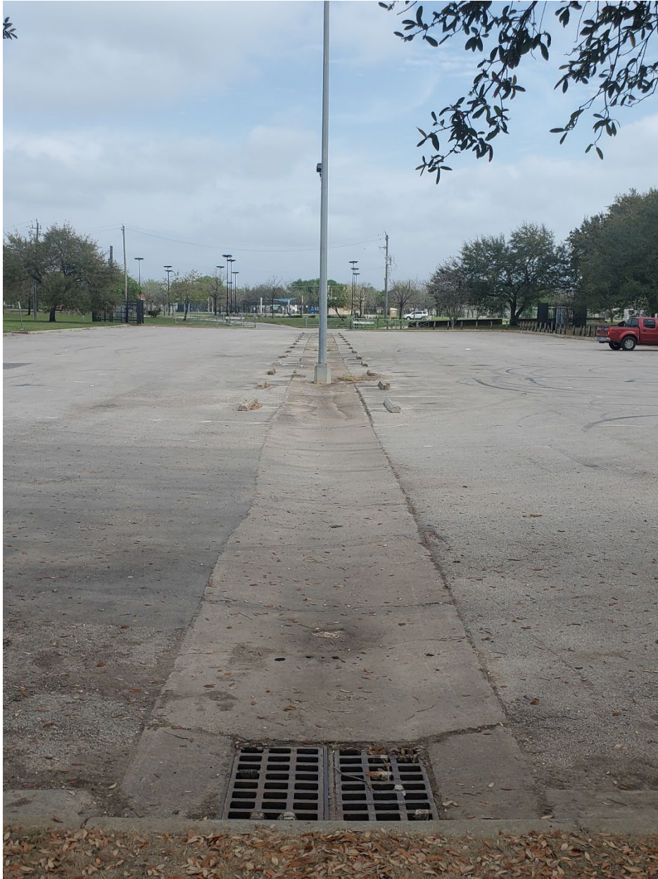
Figure 5. Image of Townwood Park concrete swale prior to construction.
