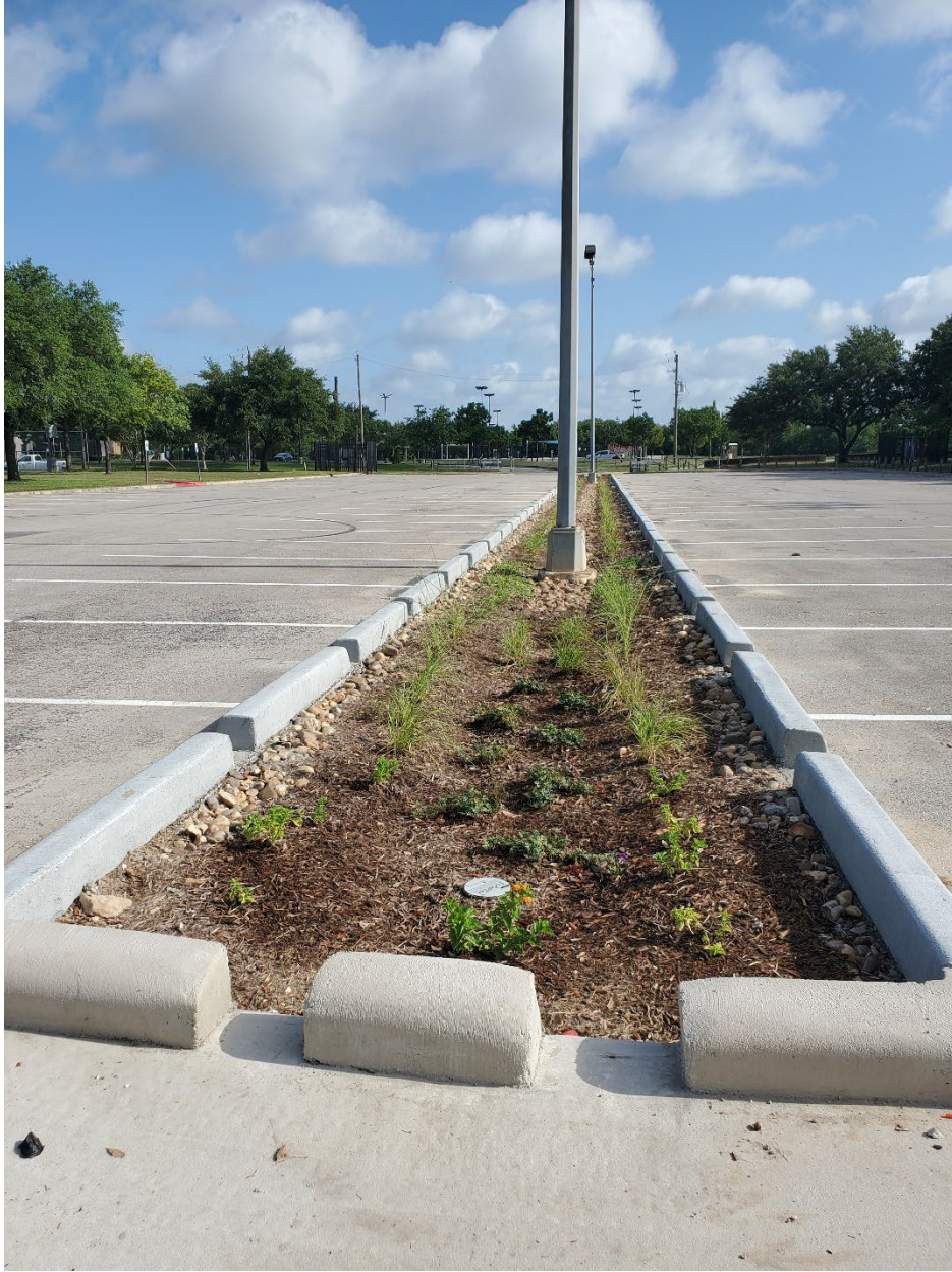
Figure 7. Townwood Bioswale after construction.
