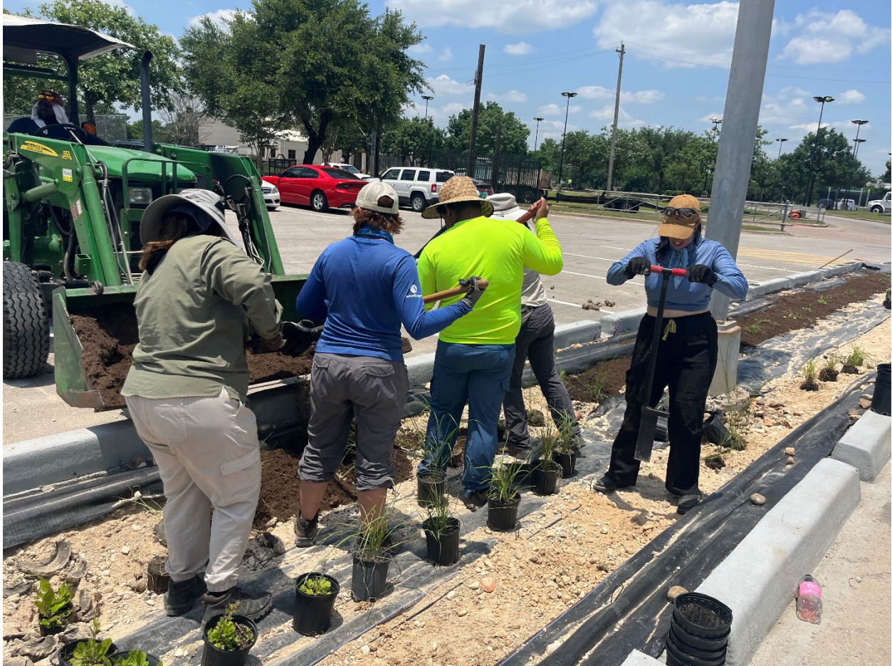
Figure 6. Townwood Bioswale during construction.
