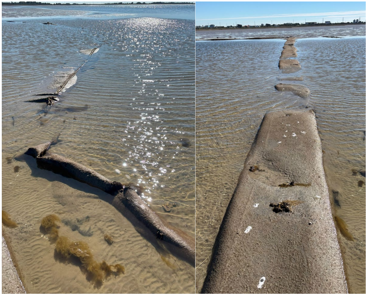
Image 1: Derelict geotextile tube within Dana Cove. at Galveston Island State Park.
