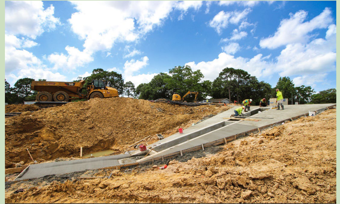
Outfall Structure, Credit: LAN, 2018
