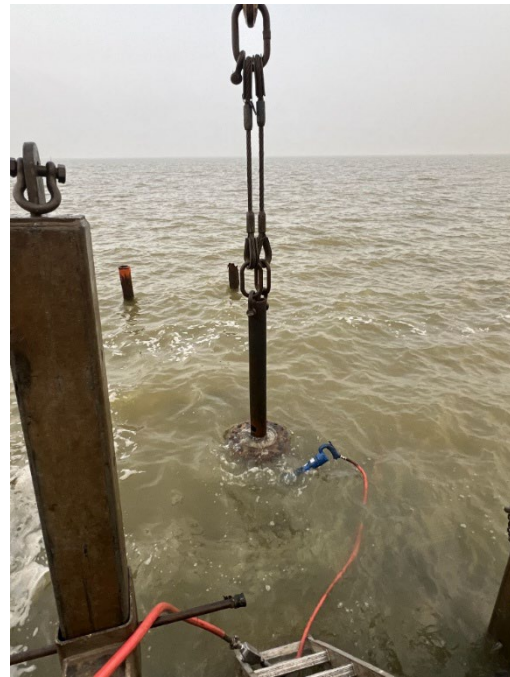
Casing Flange Underwater
