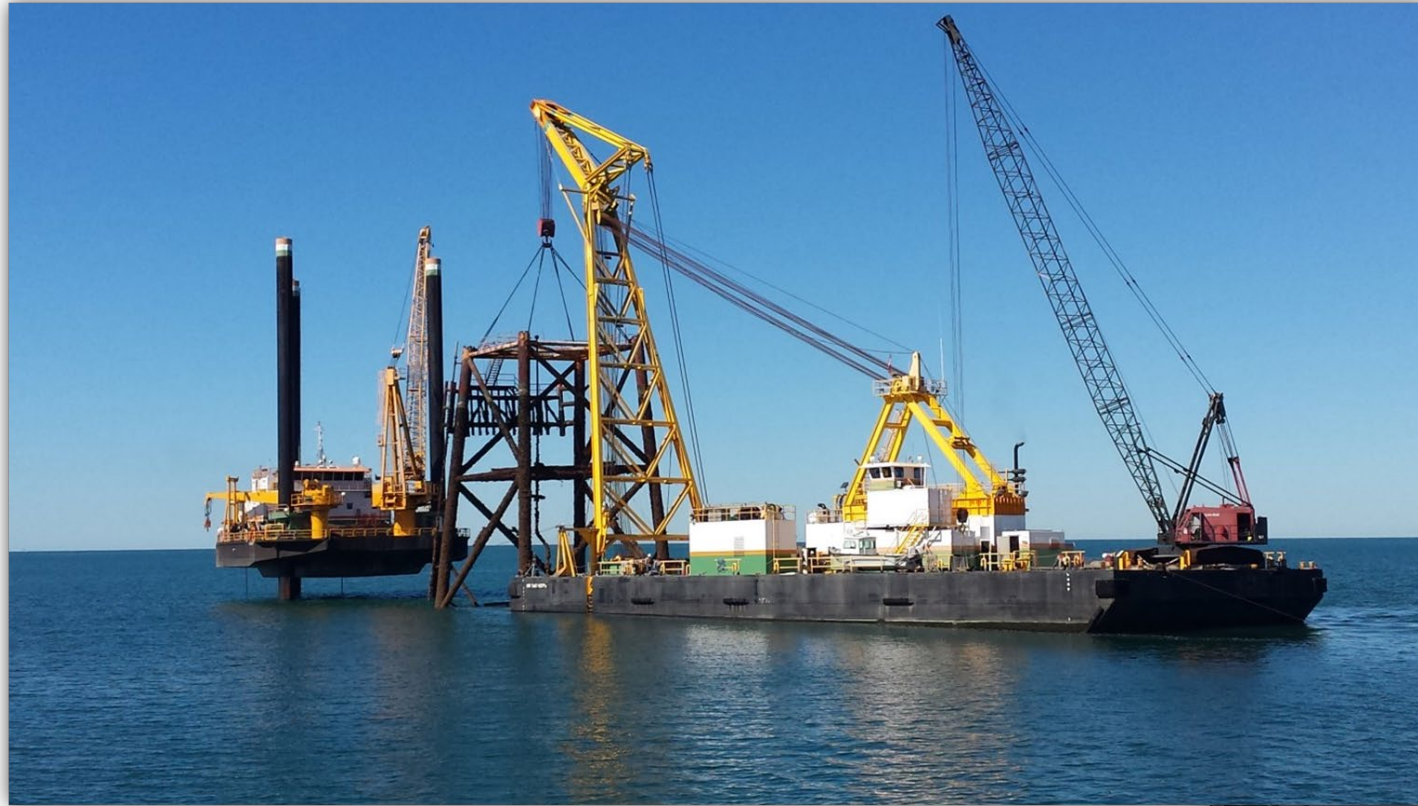
Jacket & Pile Removals
