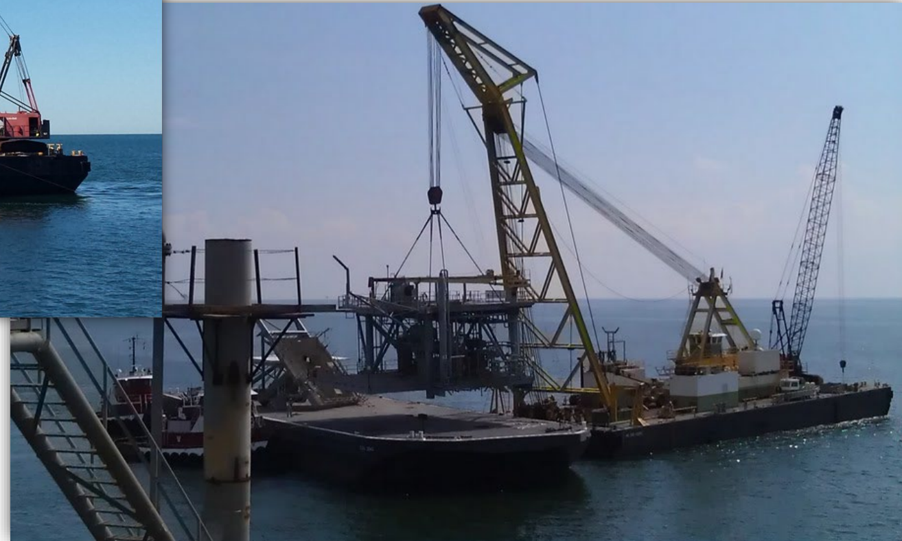
Large Deck Removals
