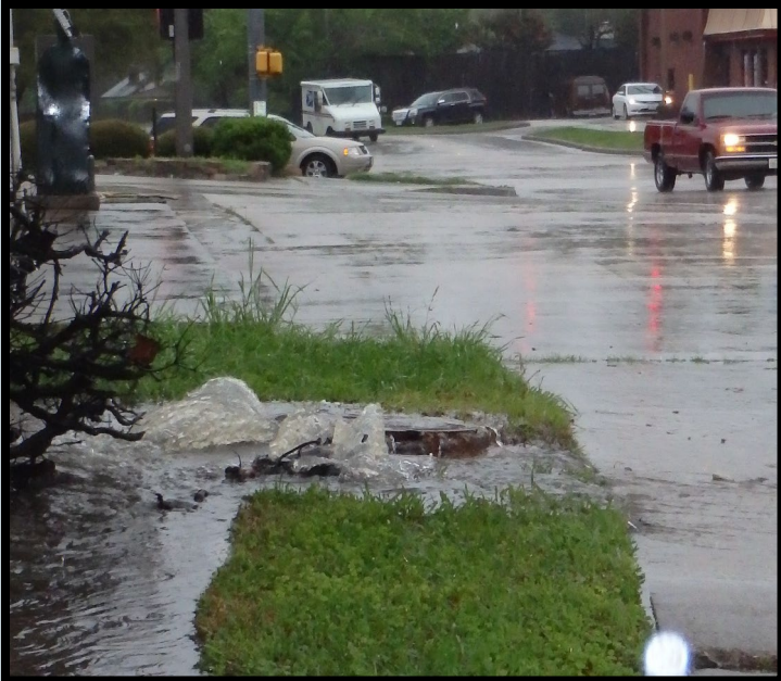
SANITARY SEWER OVERFLOWS
