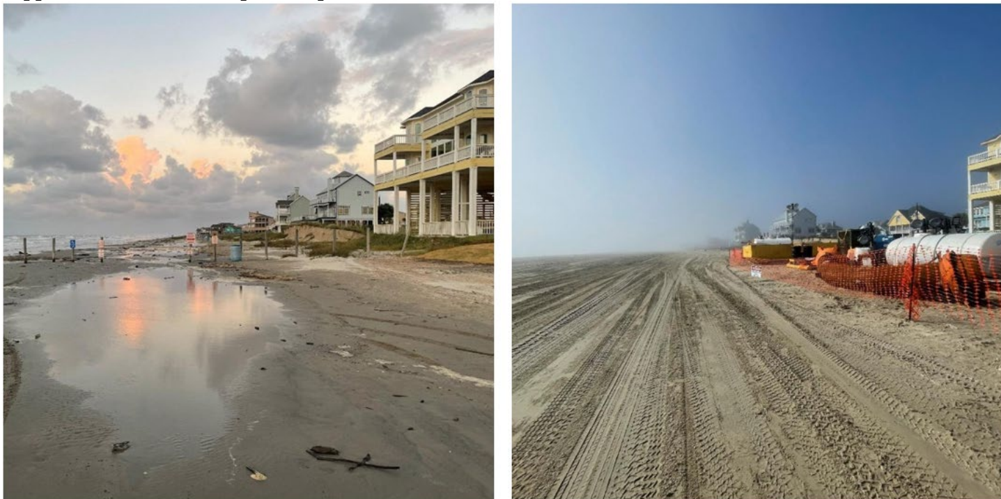
Figure 2. Beach Access #10 before and after nourishment under CAP204. The left panel shows the site prior to nourishment, and the right panel shows post-nourishment conditions following sand placement. These images illustrate the substantial physical changes in beach width, surface characteristics, and shoreline condition associated with the nourishment project.
