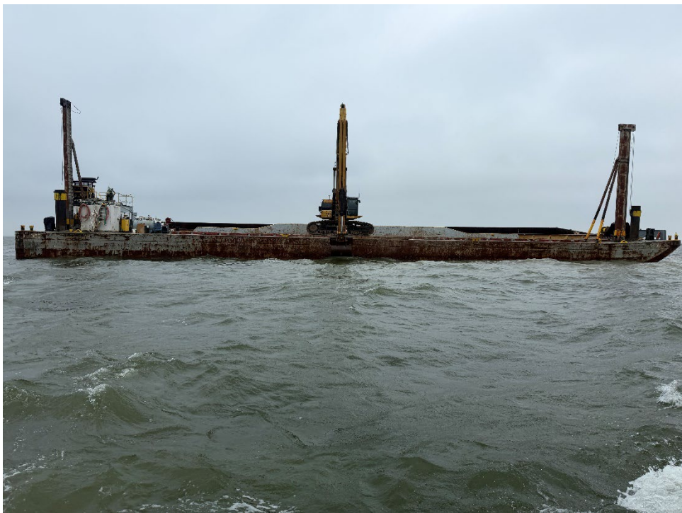
An example oyster reef restoration project completed by barge. Rock was being deployed at Beezley Reef in 2026.
