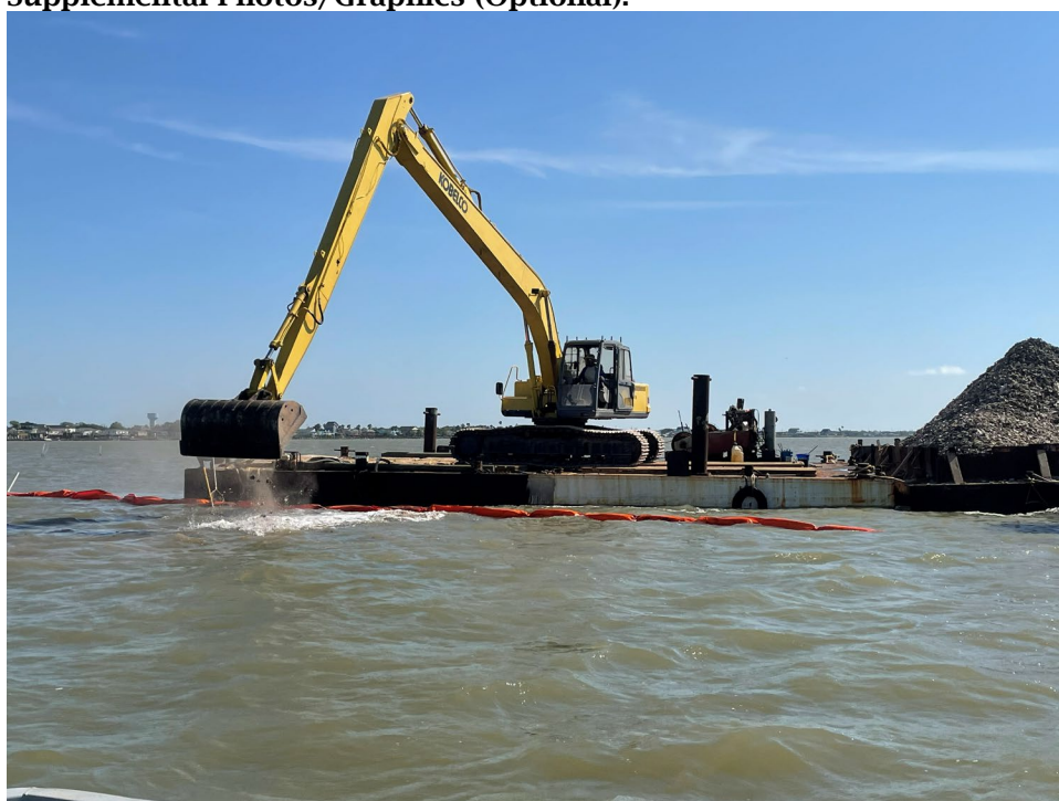
An example oyster reef restoration project completed by barge. Recycled oyster shell was being deployed at Dickinson Bay Reef in 2022.
