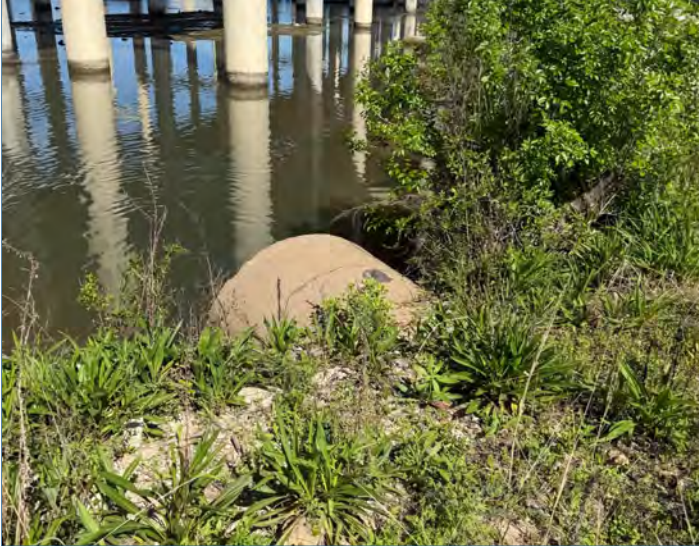
Photo 28. Downstream outfall area beneath SH 146 showing the existing pipe outlet, shoreline vegetation, and receiving-water conditions.
