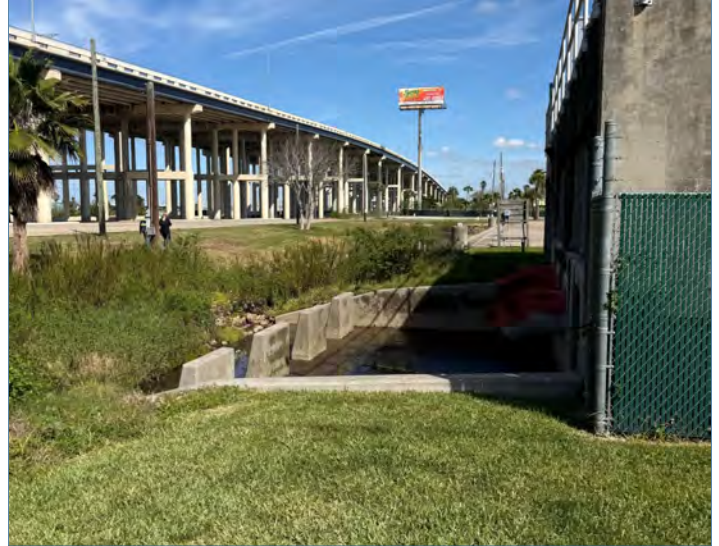
Photo 17. Pump station discharge structure and receiving channel with SH 146 immediately adjacent to the site.
