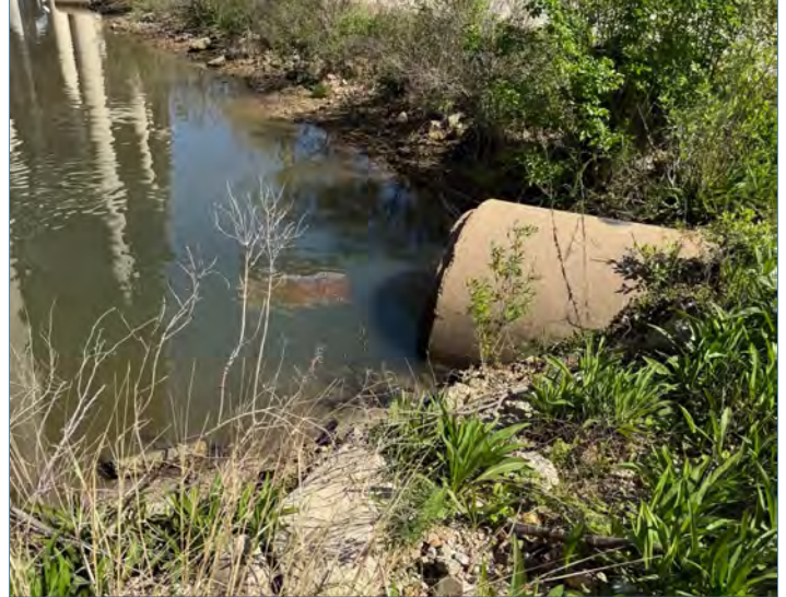
Photo 29. Additional view of the downstream outfall pipe and shoreline, documenting existing bank vegetation and receiving-water conditions.
