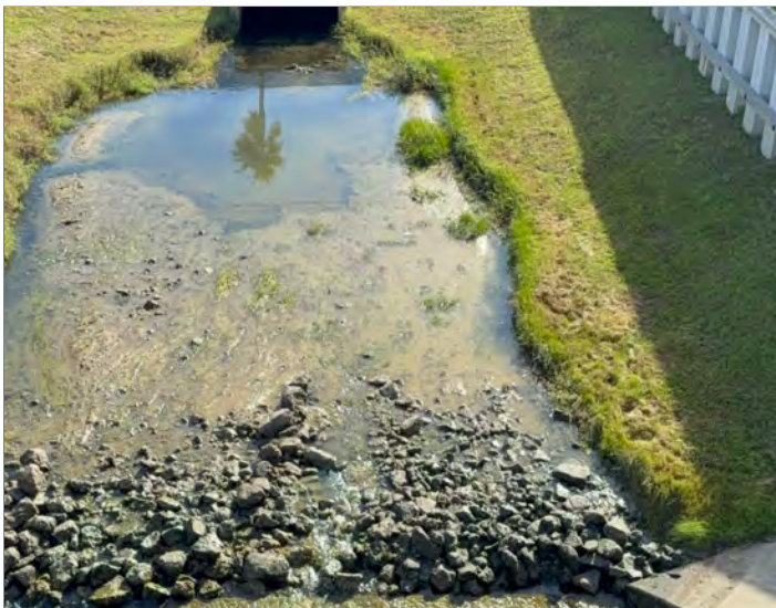
Photo 10. Existing forebay/inlet area showing standing water, exposed sediment, and the drainage box culvert.
