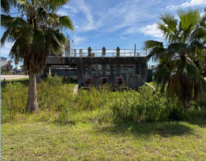
Photo 20. Exterior downstream view of the pump station structure and surrounding vegetation.
