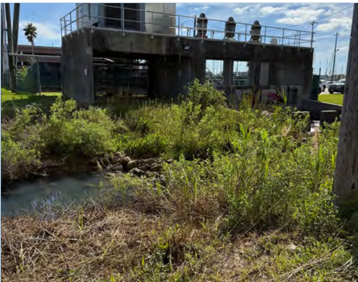
Photo 22. Pump station and receiving channel viewed from the south, showing existing channel-bank conditions.
