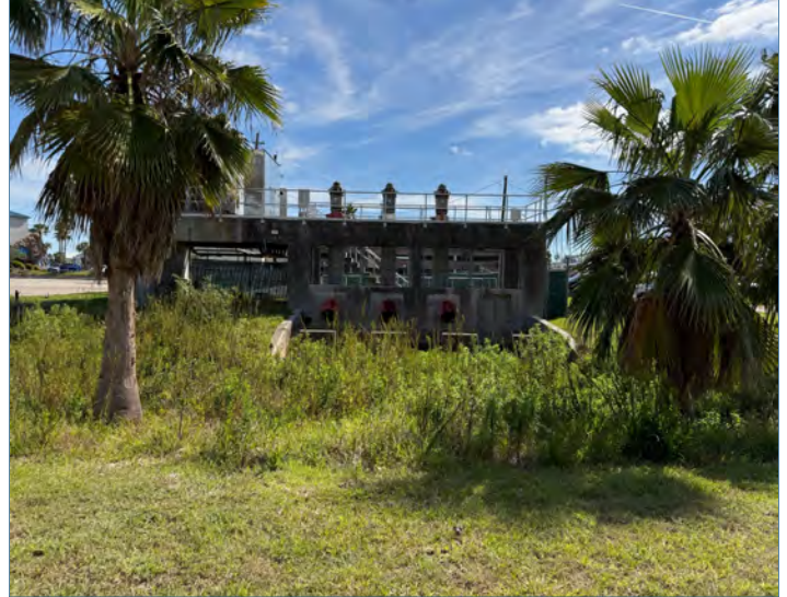
Photo 21. Exterior view of the pump station and vegetated receiving-channel area.
