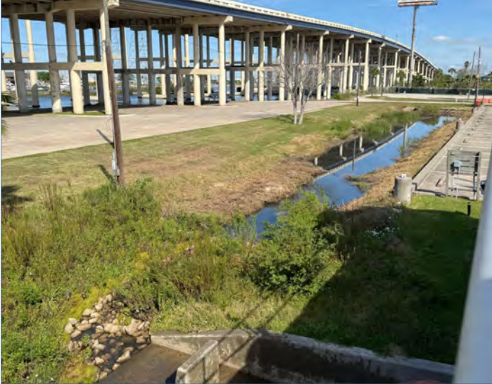
Photo 12. Receiving channel downstream of the pump station adjacent to the elevated SH 146 corridor.
