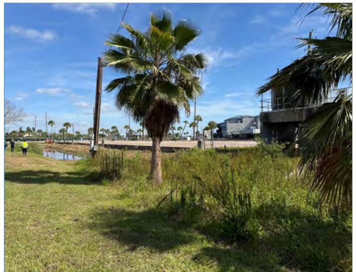
Photo 19. Existing vegetation and channel-side conditions within the proposed improvement area.
