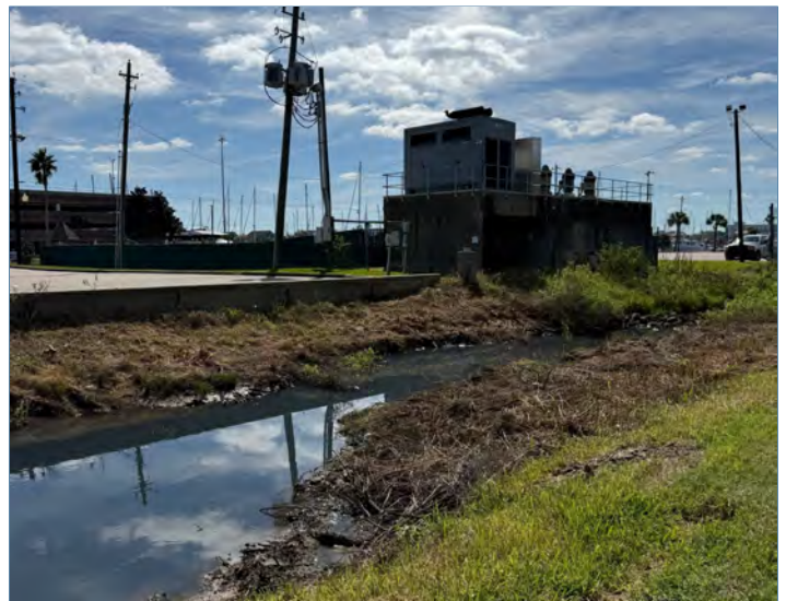
Photo 23. Receiving channel looking toward the pump station, showing existing vegetation and accumulated material.
