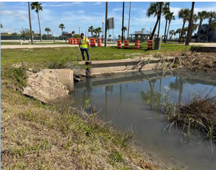
Photo 26. Existing downstream culvert/outfall area near the proposed outlet-control improvement location.
