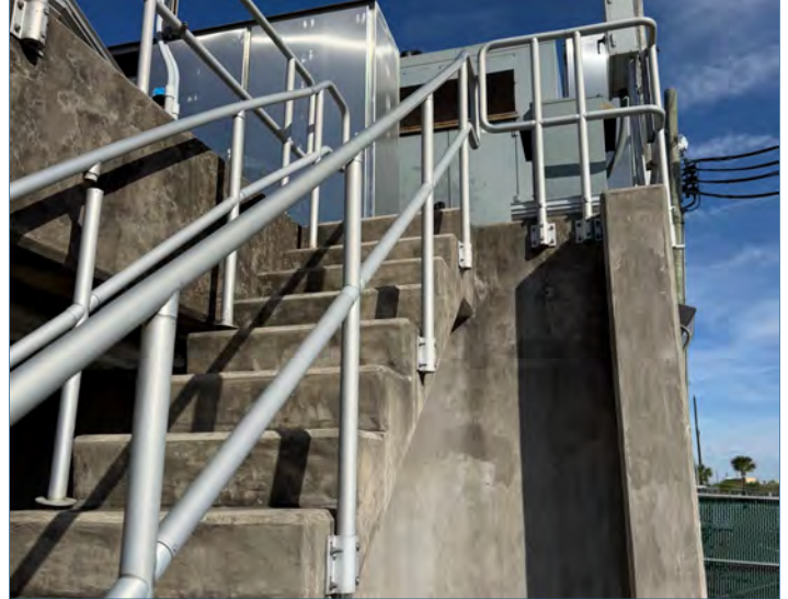
Photo 9. Existing pump station access stairs and elevated equipment platform.
