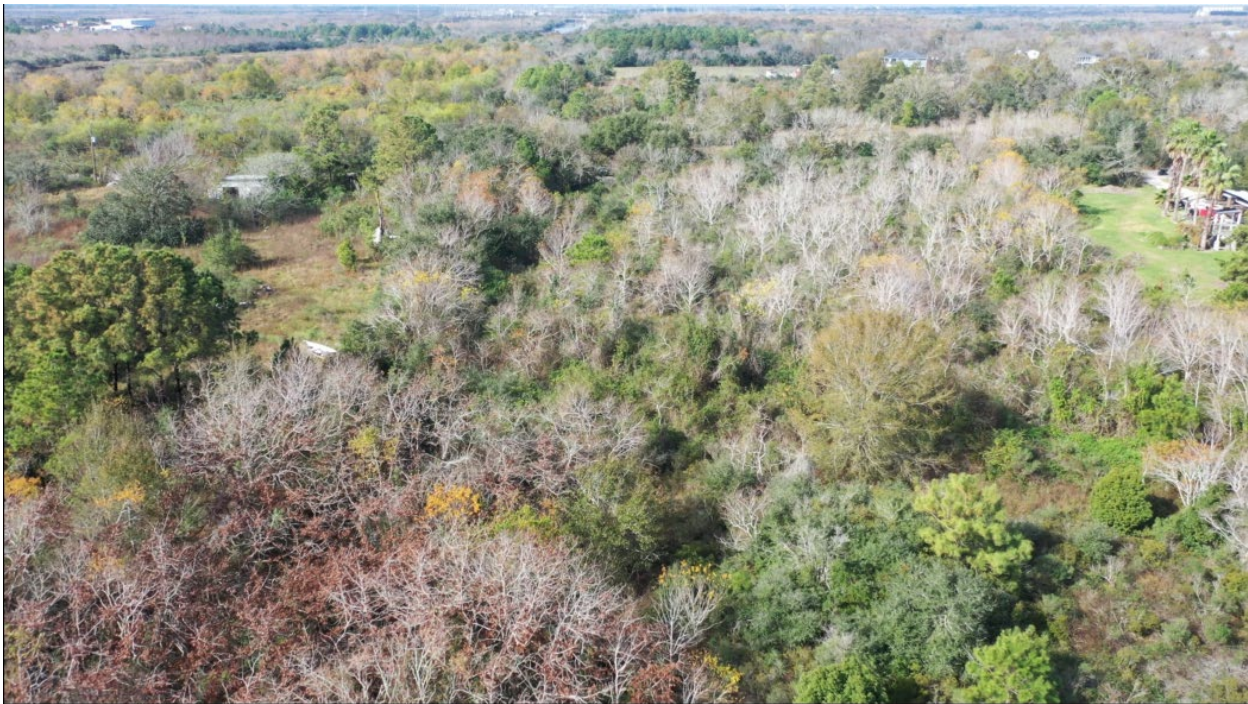
Figure 1: Salt Bayou Acquisition Project in San Leon, Texas
