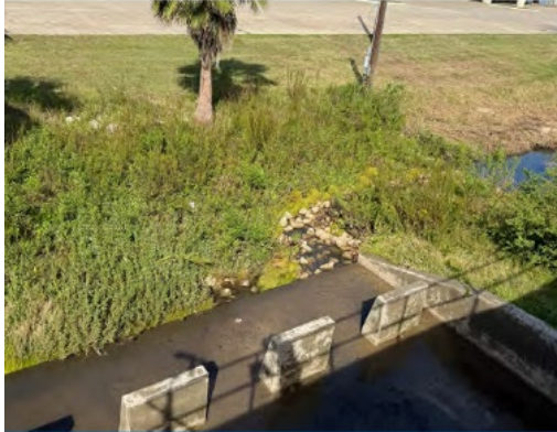
Photo 11. Pump station discharge area and receiving channel immediately downstream of the pump station.
